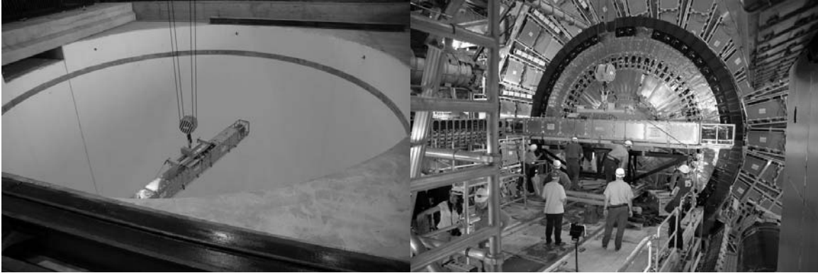
Fig. 7.7.2 (a) the pixel detector in the Dummy Support Tube (see text) being lowered into the ATLAS underground hall and (b) the Dummy Support Tube and pixel detector on a platform between the Inner Detector area and the endcap calorimeter.
